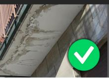
SEALIT Multipurpose is suitable for the treatment of a leaking balcony. Preparation before application is important. Remove tiles, paint and previous sealants. Ensure the area is clean and dry. Apply SEALIT to raw concrete.
