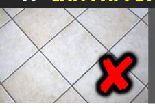
SEALIT Multipurpose is not suitable for the treatment of tiles. This sealant is designed to penetrate the concrete and block the passageway of water through fine cracks and porous sections. This is not possible on tiles.
